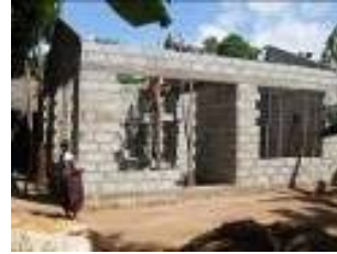
House at Sooriyawewa (Now completed)
